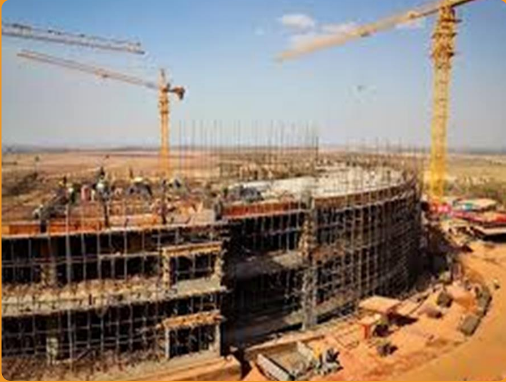
“A typical construction site”
